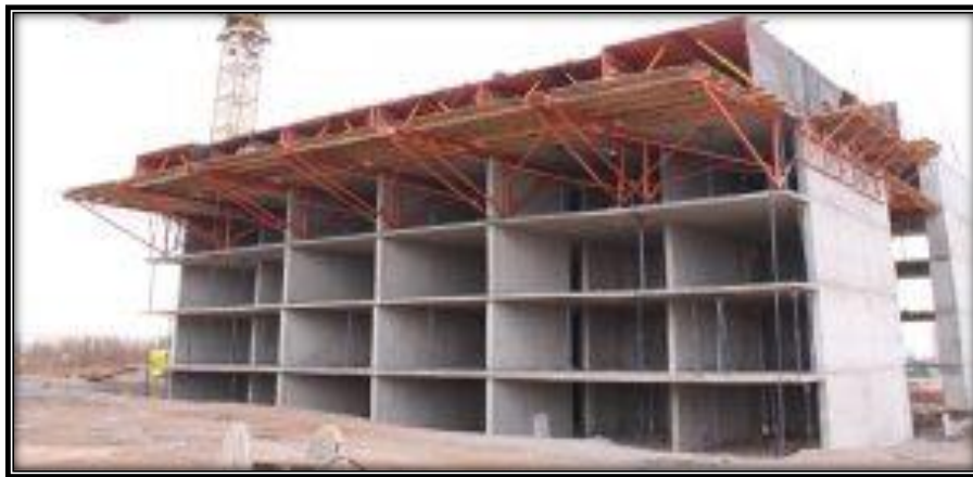
(fig.24 Tunnel Formwork System)
