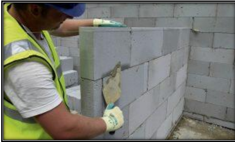
(fig.27 Thin Joint Masonry Technique )
