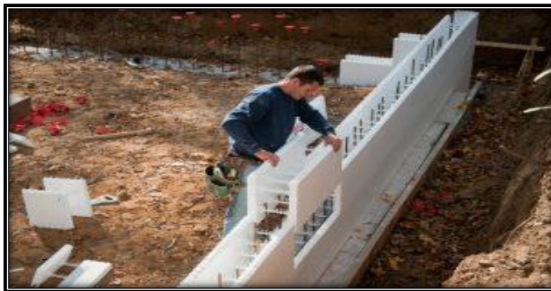
(fig.28 Insulating Concrete Formwork (ICF) Technique)
